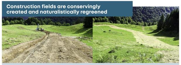
The strips of sod, such as here for the artificial snow technology systems at Burgstall, are carefully removed, stored sideways and then replaced. Sowing takes place with indigenous, species-rich seed mixtures (nutrient-poor grass, species-rich extensive meadows, etc.). The seeds are covered by indigenous hay mulch and is therefore able to develop nicely under moist and protected conditions. Furthermore, this kind of rapid regreening also ensures that grazing may take place.
